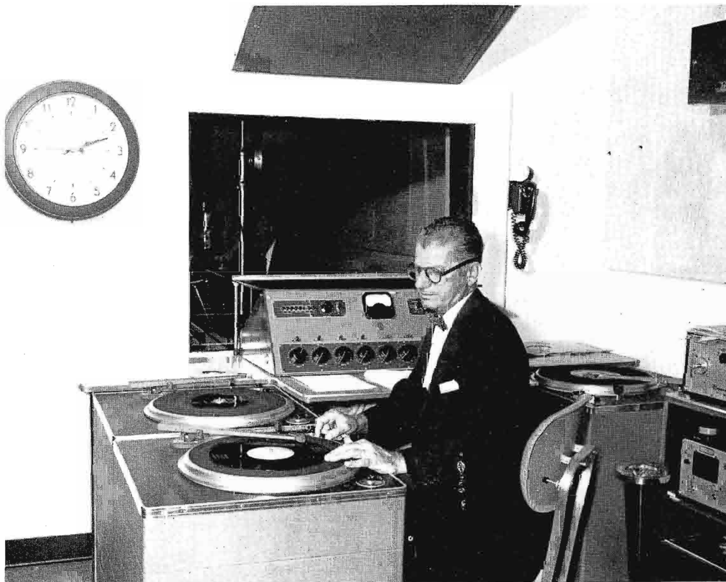
FIG. 7. Studio "B" control room is typical of the facilities available in the other two control rooms and contains a BC-2B Studio Consolette, three BQ-2A turntables, tape recording equipment and LC-1A monitor loudspeakers.
