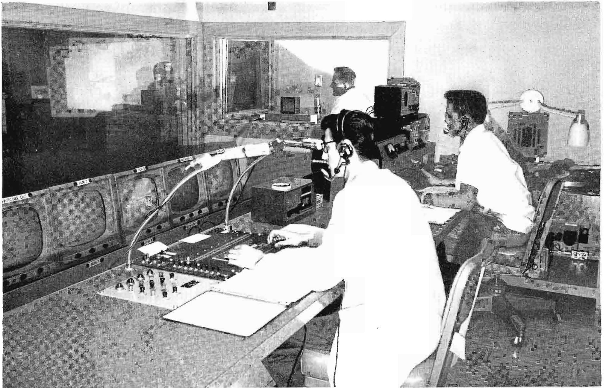
FIG. 13. View of studio "B" production control with announcer's booth in the background. Desk equipment in this control room is similar to that of control room "A", permitting familiarity when operators and directors switch from one room to the other.
