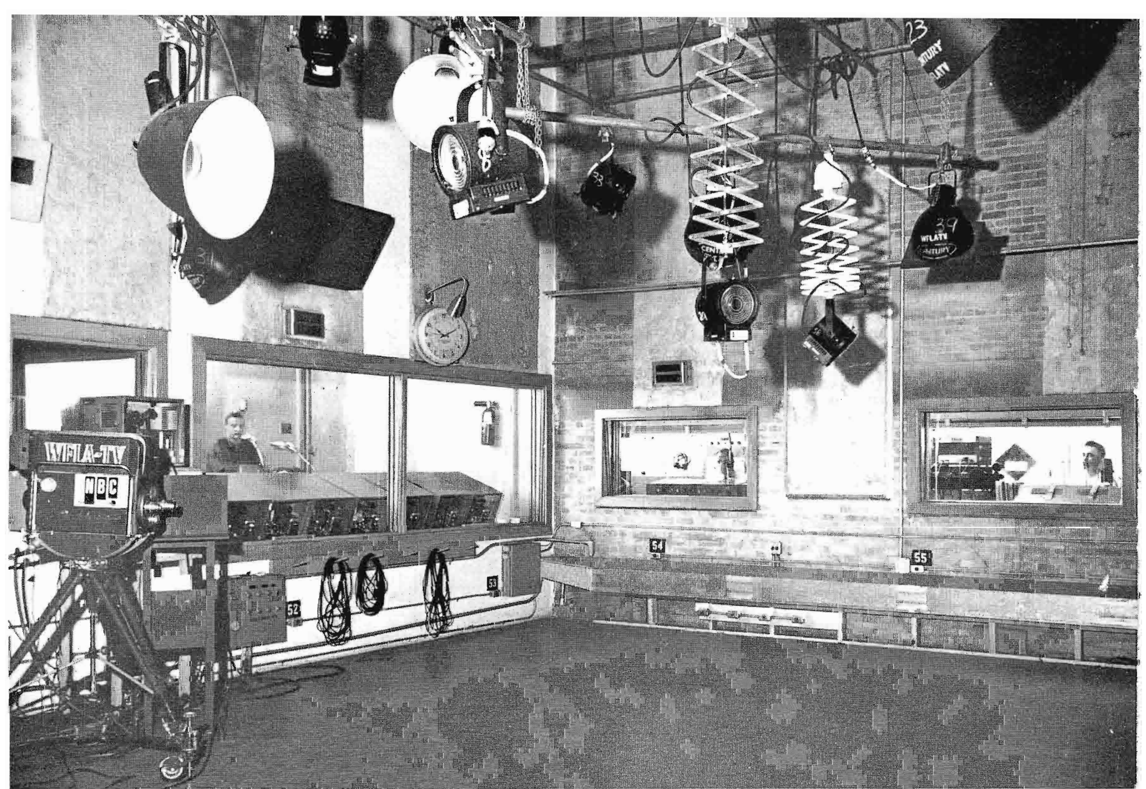
FIG. 11. Studio "B" showing both television and radio control rooms. The small window on the left behind the camera is "H" Announce Booth. The large window to the left of center looks into "B" studio television production control room. The smaller window just to the right of television control room looks into radio control with an RCA 76-C audio console and rack equipment in the background. The window on the extreme right looks into radio announce booth with an RCA BC-2B console. A 44BX mike and a tape recorder being visible in front of the announcer. "On Air" lights above each of the television and radio control room windows are operated from their respective control points. There are microphone outlets in this studio from both television control rooms as well as radio control.
