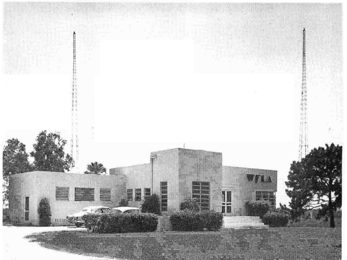
FIG. 33. View of the front of the AM transmitter building with the three-tower directional array in background. Building was constructed in 1940.
