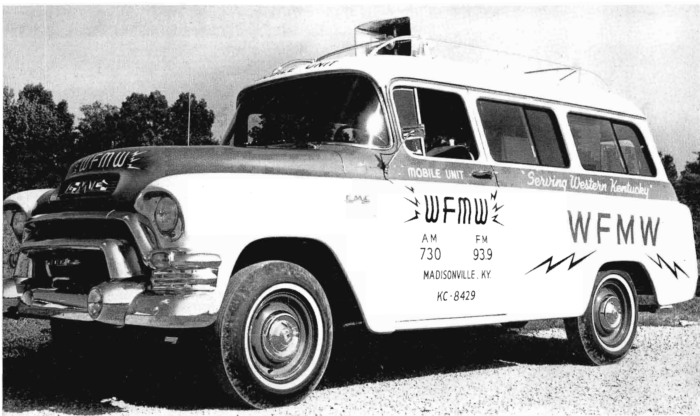
FIG. 1. Mobile unit remotes are relayed to station via 450-mc broadcast relay band.
