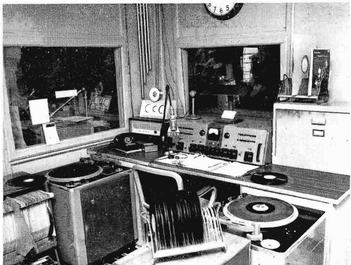
FIG. 5. Main control room showing the "Carfone" receiver just to the left of the studio console. Main studio can be seen through the window in front of the operator.
