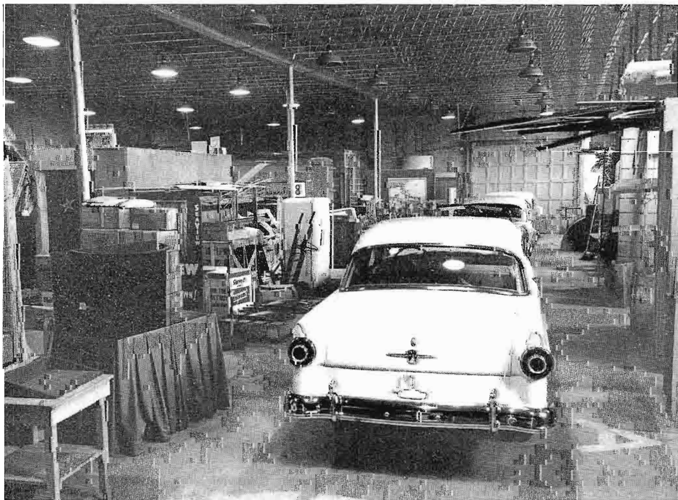
FIG. 12. Property room showing auto drive-in door at rear.
