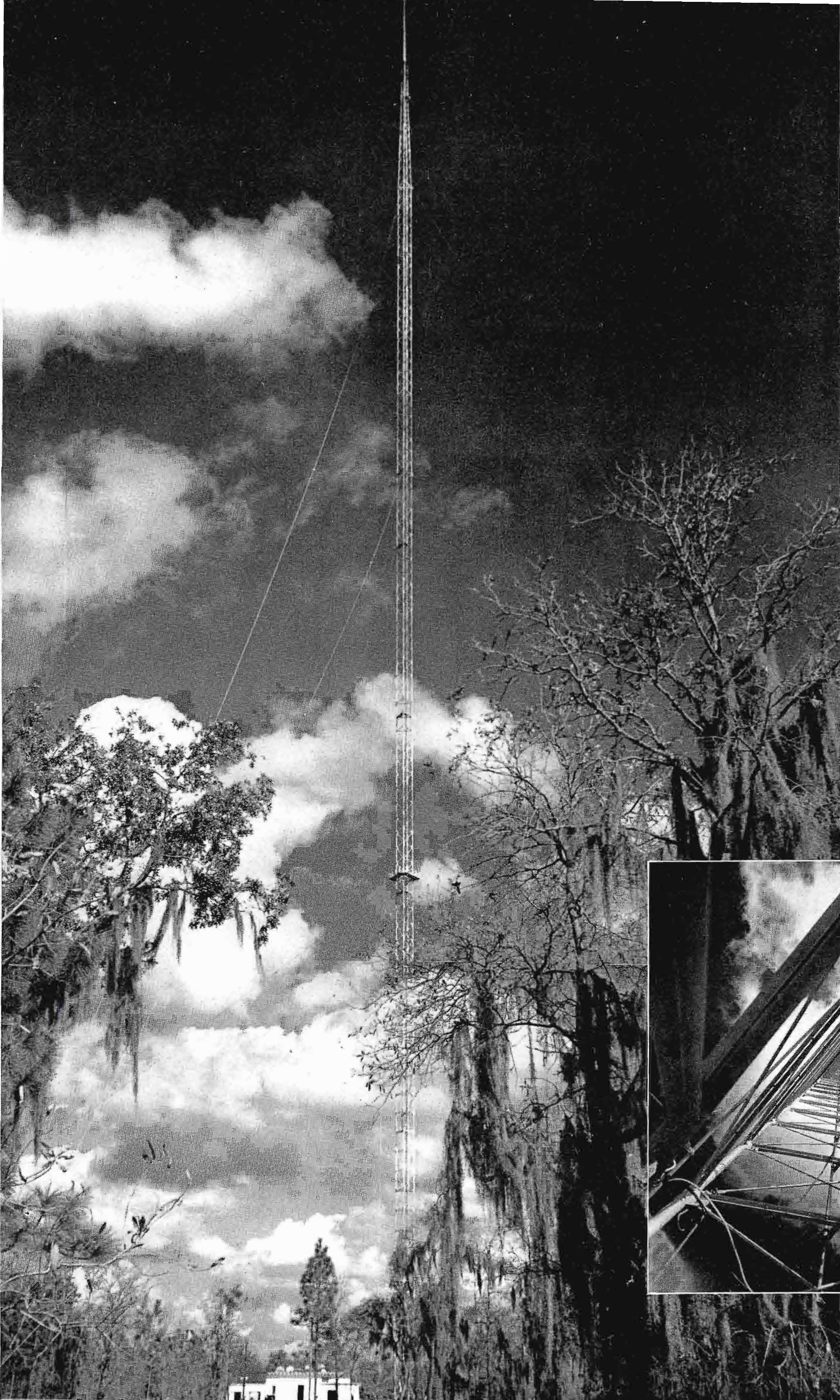
FIG. 25. WFLA-TV tower and antenna point 1055 ft into Florida skies. The Ideco tower structure supports an RCA TF-12AH twelve-section superturnstile antenna. Looking through a picturesque setting of trees bearing Spanish Moss, the transmitter building is visible at the base of the tower.
